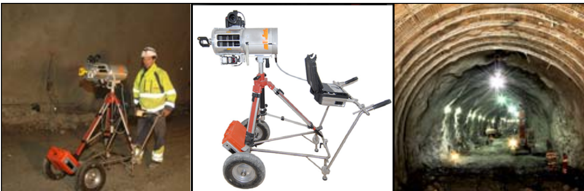
Figure 1: Data acquisition platform equipped with laser scanner and camera (left, center), tunnel site(right)
